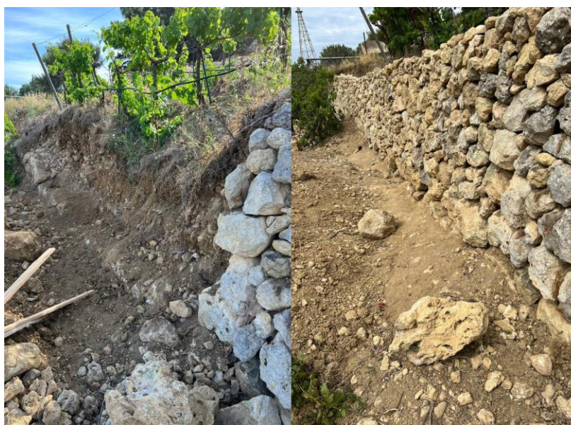
Before and after rubble walls restoration works
