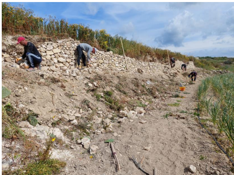
The rubble walls restoration works in Manikata
