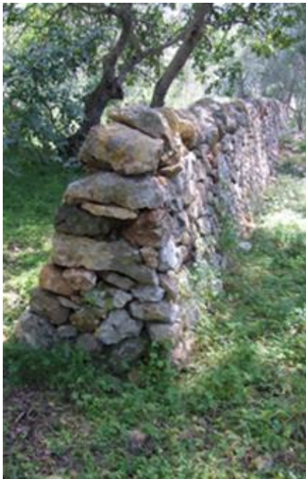
Fig. 8 – Rubble wall with tapered structure
