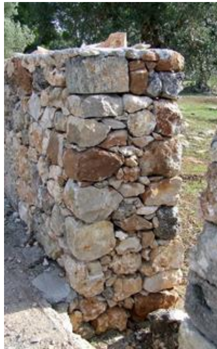
Fig. 9 – Rubble wall with parallel sides
